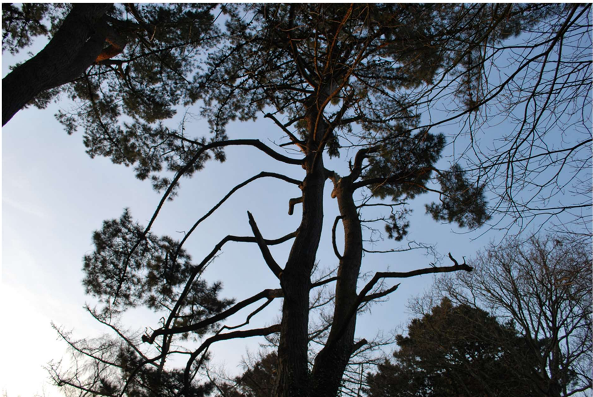
Overall poor quality of tree from past poor pruning and failures
